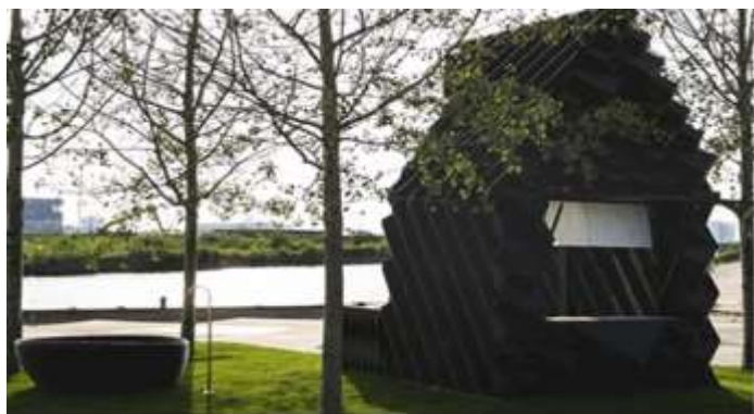
Figure 8 (a) shows the first 3D-printed home by DusArchitects [257] and (b) shows a 3D-printed home by WinSun [3].
